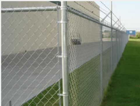
Galvanized Chain Link Fence
