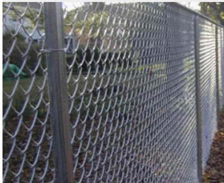
Galvanized Chain Link Fence
