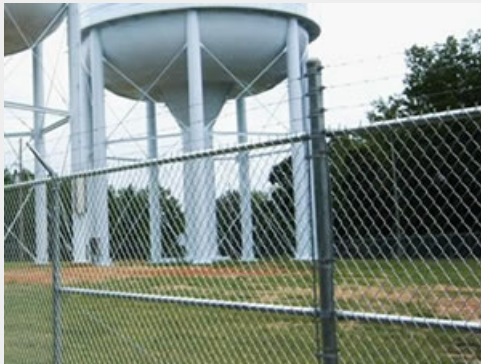
Galvanized Chain Link Fence
